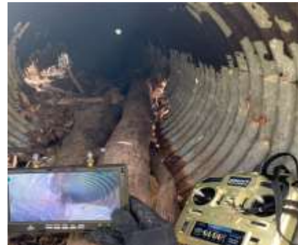
a. b. Figure 1 Small culvert with difficult access for humans: a. Exterior entrance, and b. Inside view with other entrance visible [5].
