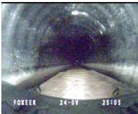
Figure 5 Example sensing options: a. FPV camera view from inside culvert [5], and b. Mechanical tapper with digital microphone for bridge deck sensing undergoing laboratory tests.
