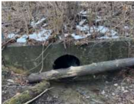
a. b. Figure 1 Small culvert with difficult access for humans: a. Exterior entrance, and b. Inside view with other entrance visible [5].
