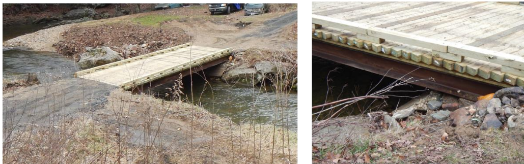
Figure 3. Typical temporary bridge built after Hurricane Helene in Wester
