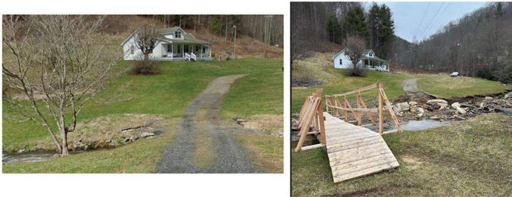
Figure 2. Local Crossing (PO141) in Creston, NC, 377% Channel Width Widened
