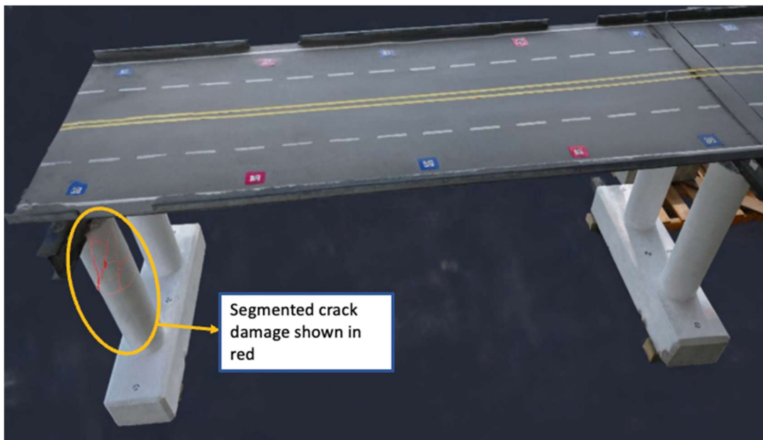
Figure 3: 3D mapping of the segmented cracks
